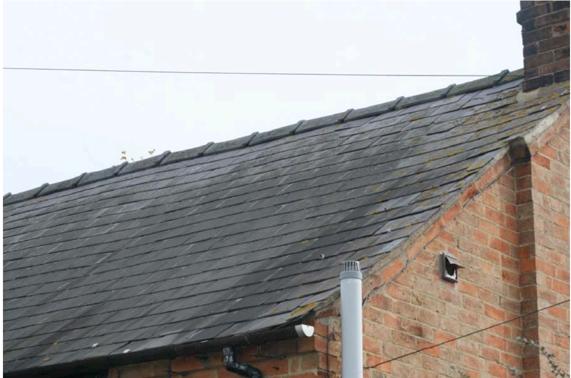
PHOTOGRAPH NO. 1 Front face of main roof
