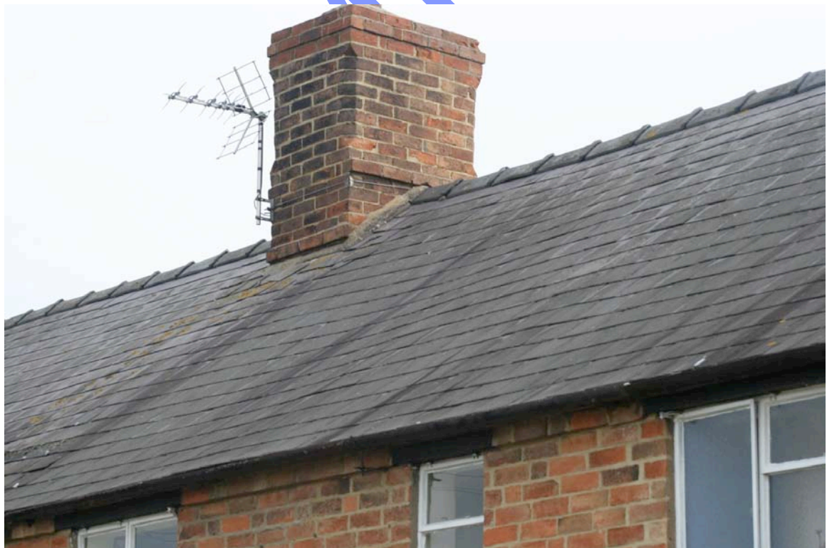
PHOTOGRAPH NO. 2 Front face of main roof
