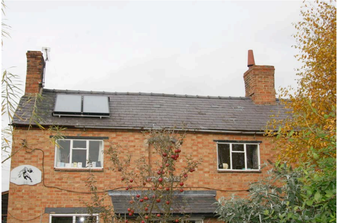
PHOTOGRAPH NO. 5 Rear face of main roof
