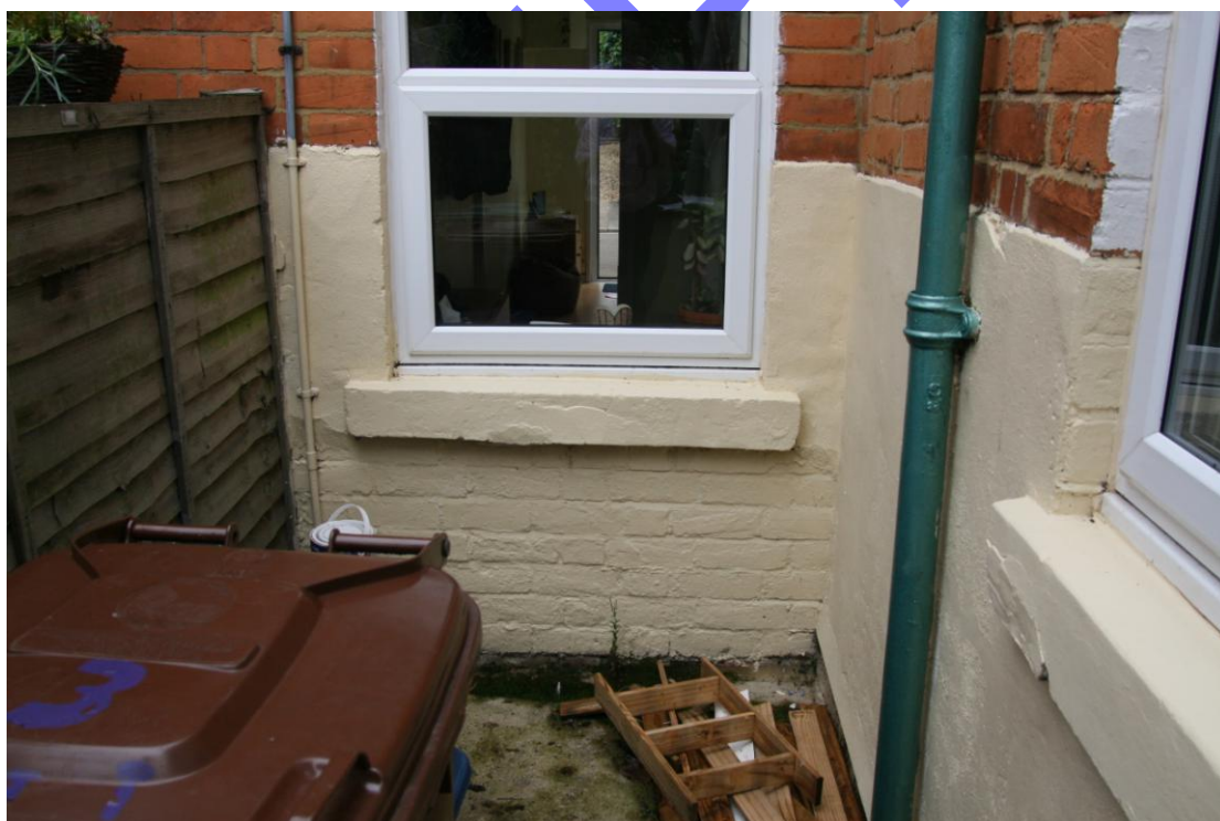
PHOTOGRAPH No. 9 - Distortion in the window openings
