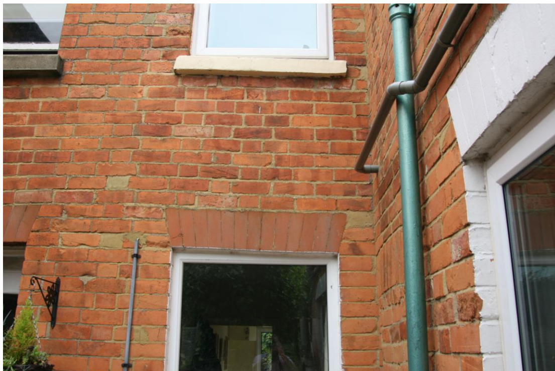
PHOTOGRAPH No. 9 - Distortion in the window openings
